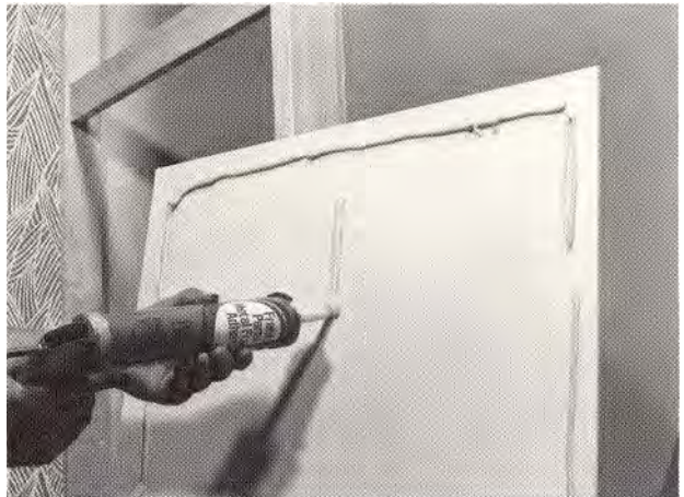
Apply adhesive to ceiling panels
