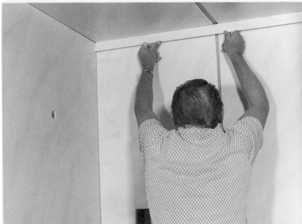
Install ceiling trim
