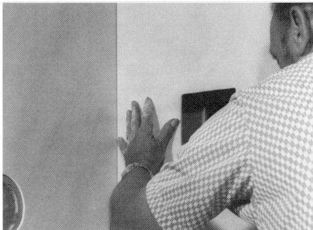
Leave 1/8" gap in corners for caulking
