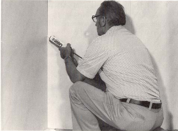
Caulk all joints, corners and edges
