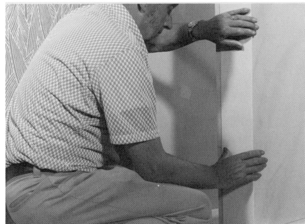
Install Corner trim
