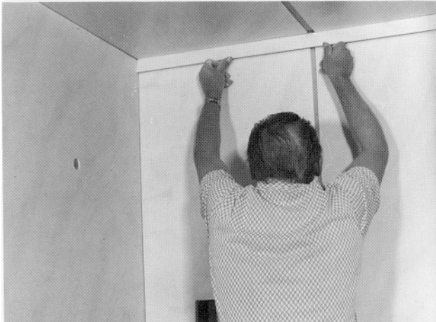
Install ceiling trim
