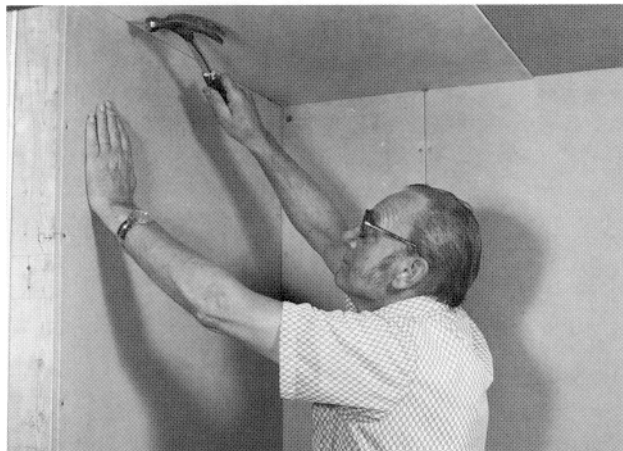
Cut and install ceiling panels
