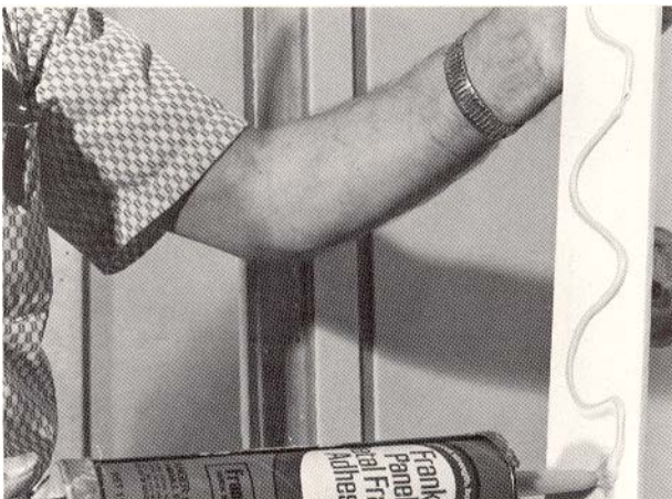
Install casing strips
